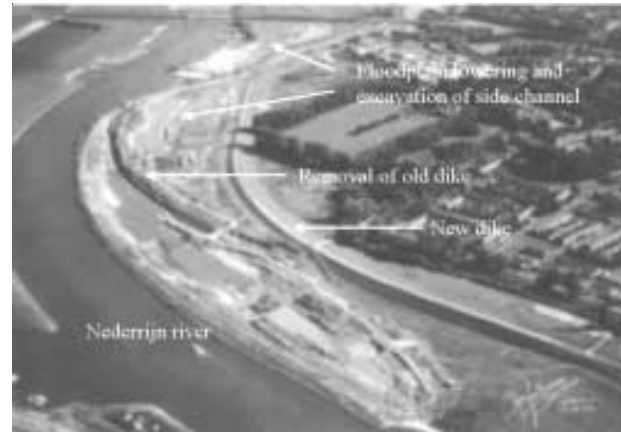
Figure 3. River dike relocation, creation of side channel, and floodplain lowering in Bakenhof along the Nederrijn river at Arnhem. For details on the efficiency of this project see Tables 1 and 2
