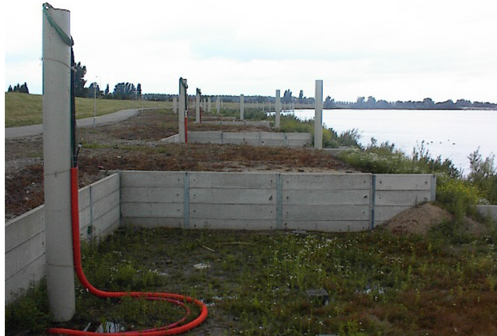
Flexible facility connections between two houses, before connection to the house.
