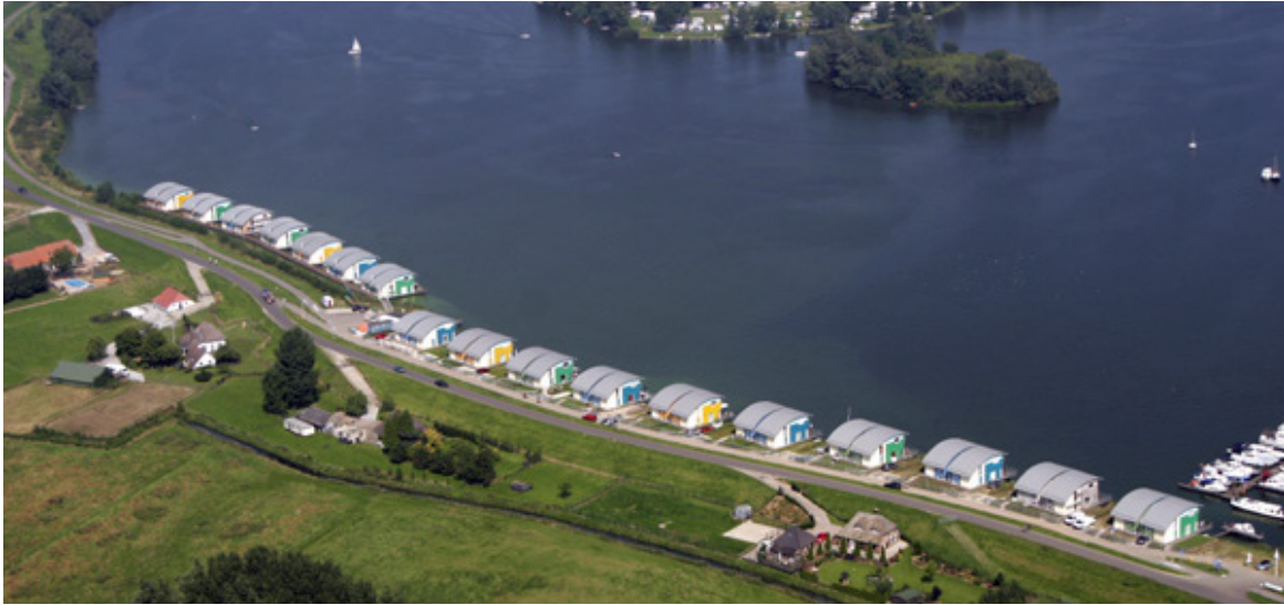
Floating and amphibious houses with access road and floating pier. (image: studio van hesse)
