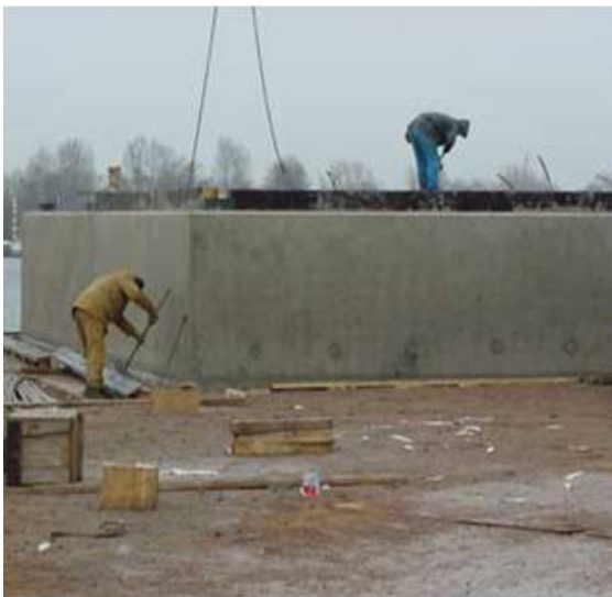
Prefabrication of concrete hulls on site.
