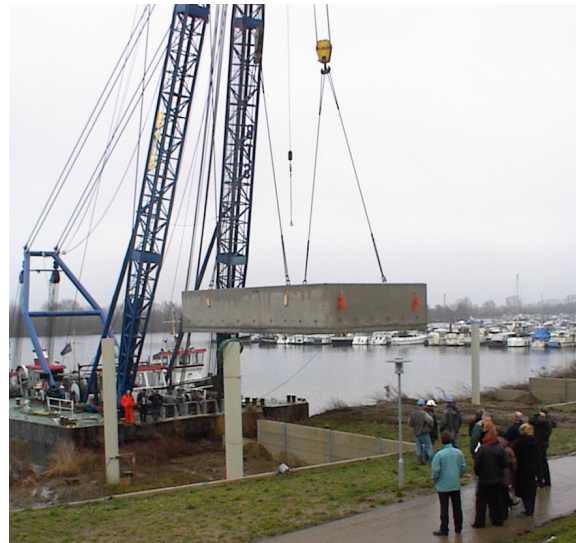
A concrete hull is hoisted from the water into the dock of a amphibious home.
