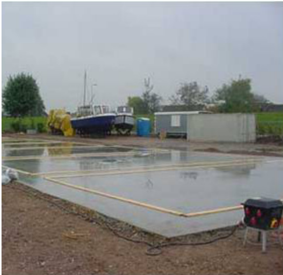
Prefabrication of concrete hulls on site.
