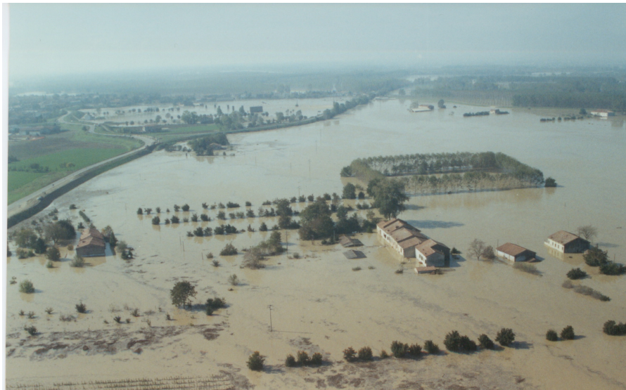
Figure 6 Main embankment along the Po River, in the vicinity of the town of Agoiolo.
