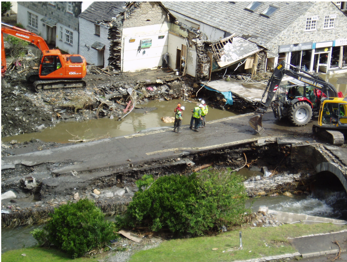
Figure 1 Flood damage at Boscastle UK (courtesy HR Wallingford).
