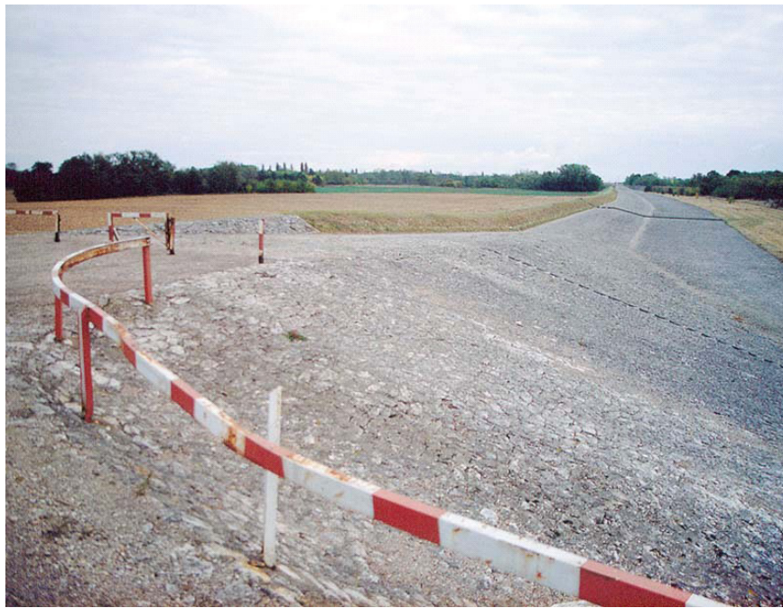
Figure 2 Spillway in Middle Loire embankment (courtesy HR Wallingford).
